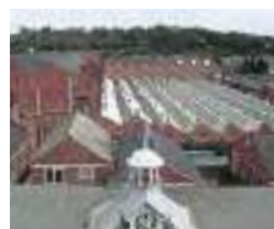
NSK Newark Plant
